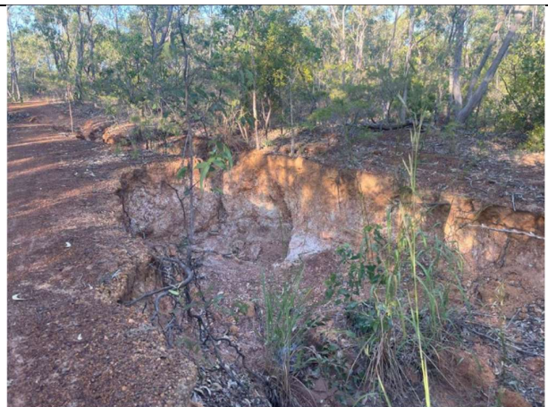
Figure 2-2 – Erosion Gullies Example 2
