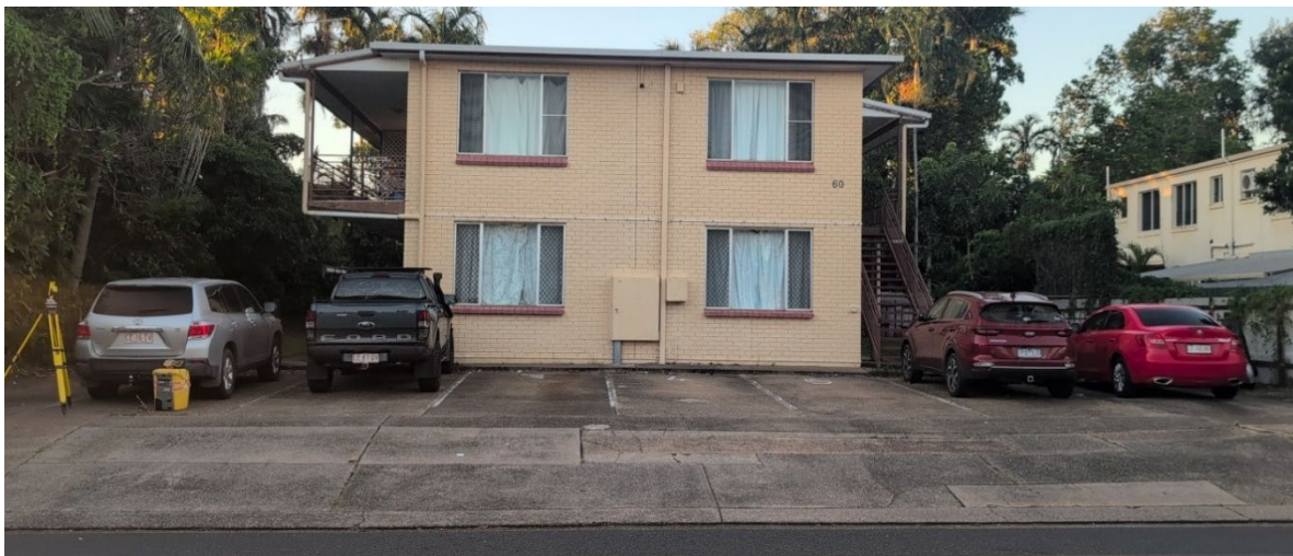
Image 6: Existing Progress Drive interface at 60 Progress Drive, Nightcliff.
