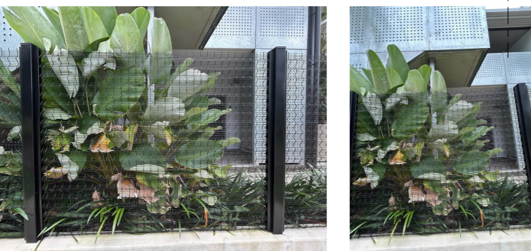
IMAGES OF 1500mm HIGH ANTICLUMB FENCE TO FRONT BOUNDARY (FACING PROGRESS DRIVE)
