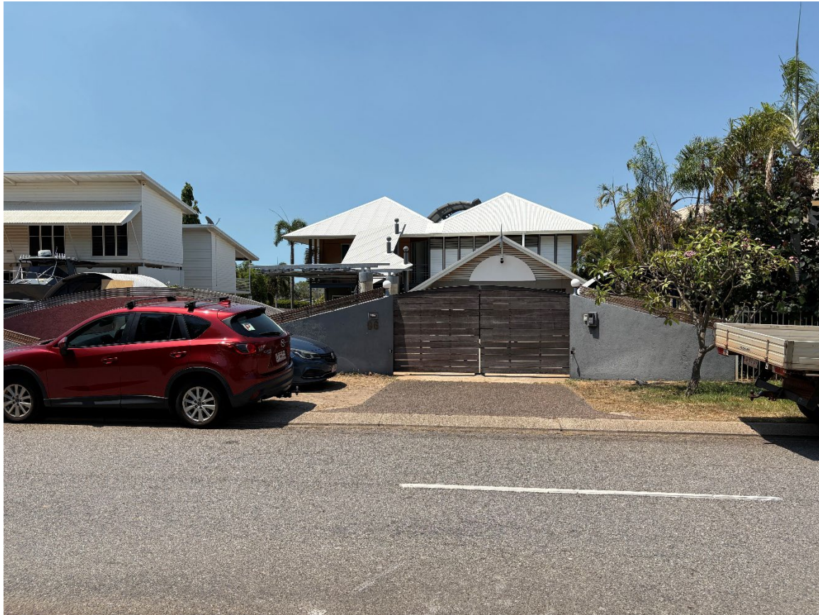
Figure 1 – Existing dwelling from Cullen Bay Crescent
