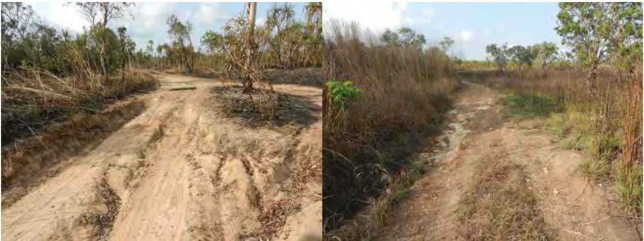
Figure 10: Examples of erosion within the site
