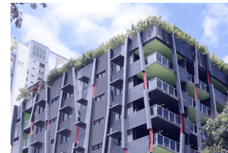
Fig 6: Rooftop planting can reduce heat absorption from the sun and provide natural cooling.
