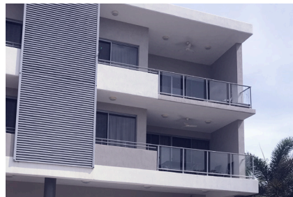
Fig 3: mixed permeability balustrades provide a balance of view out, while restricting views in.
