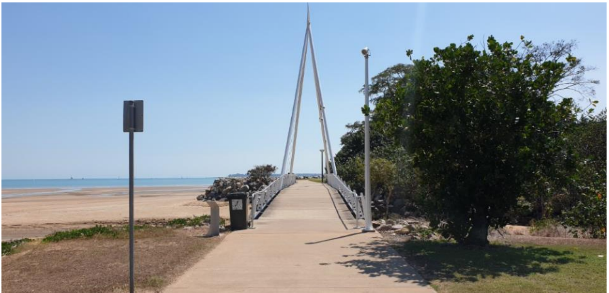
Image 6: Pedestrian bridge over mouth of Little Mindil Creek
