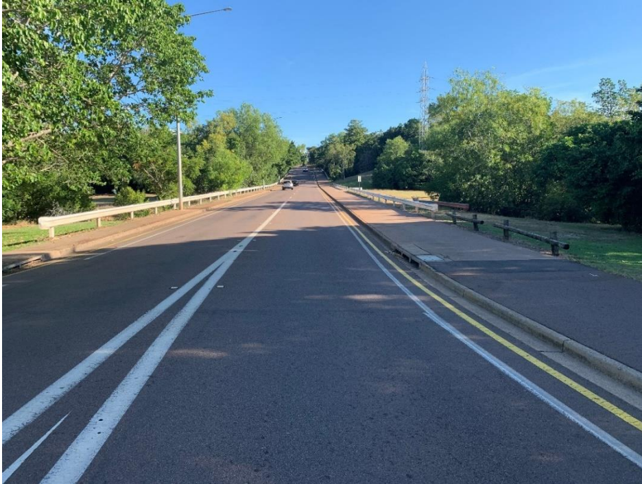
Figure 3- Existing shared path next to the subject site
