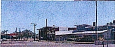
Humpty Doo Police and Fire Station
