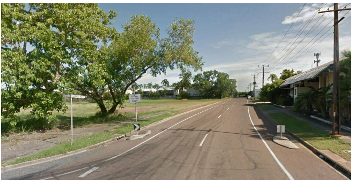
Figure 9b : Existing condition of verge on west side of Gardens Hill Crescent
