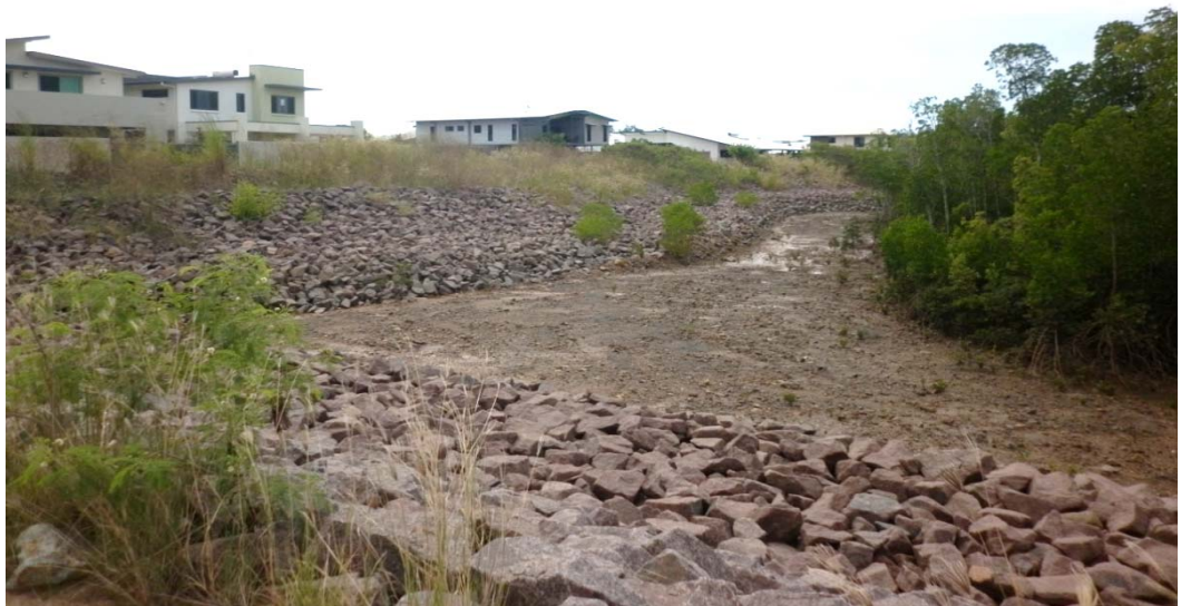
Plate 2: View of existing embankment and site surface at Lot C
