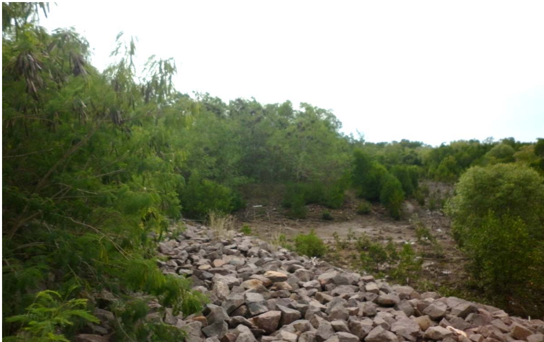
Plate 1: View of existing embankment and site surface at Lot A
