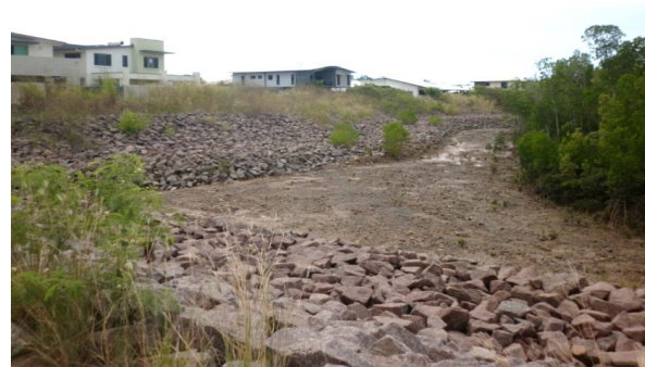
Plate 2: View of existing embankment and site surface at Lot C
